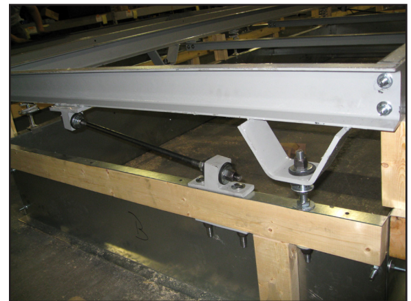
Vertical and Horizontal Seismic/Wind Restraints. Meets the current IBC Building Codes
