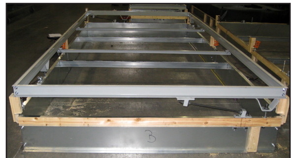
Flexible Supply and Return Duct Support Hardware Installed
